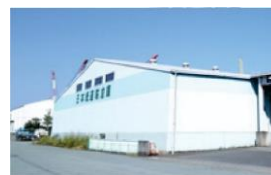
Yatsushiro No.5 Warehouse
